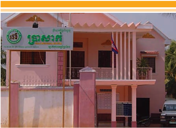
PRASAC branch office in Kampong Chhnang province, Cambodia
